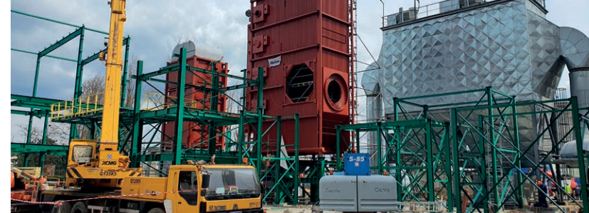
↑ New cogeneration unit construction at Expur site in Slobozia (Romania)
